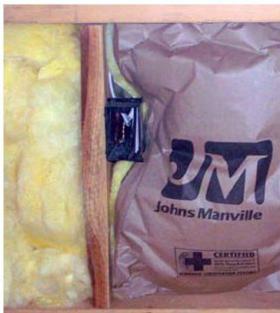
Above left: Cut fiberglass batt insulation to fit around electrical boxes, wiring and pipes that run through the walls. Compressions like the one shown above can ruin the batt's thermal alignment with the wall, which decreases its effectiveness.
