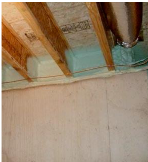
Above: Spray foam along the basement rim joist to provide a complete air barrier connecting the foundation wall, sill plate, rim joist and subfloor (Source: BSC, 2009).
